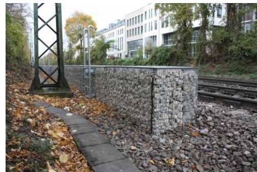
Figure 1. A gabion wall installed as noise barrier next to a railway track (source: www.heringinternational.com).
