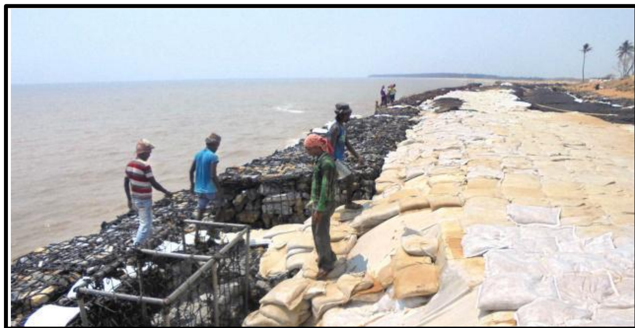
Geo – Synthetic Tube at Pentha village in Kendrapada District
