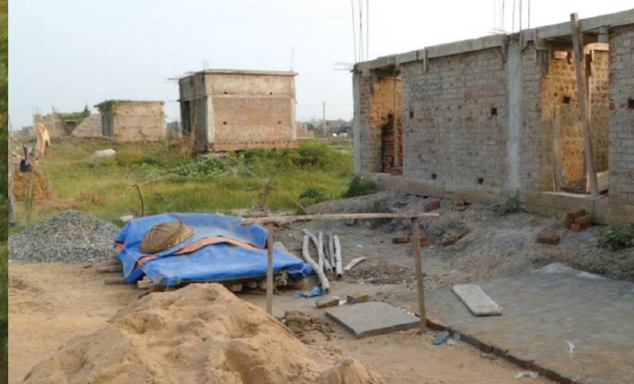
Houses under construction in Bagapatia.
