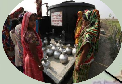
pond sand filters
