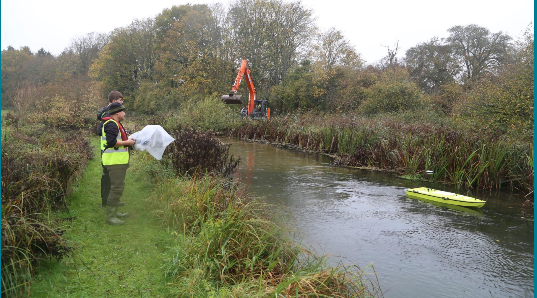
Remodelling the hydraulics of the Oakley Beat on the River Test
