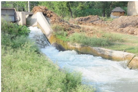
Fig. 4: Typical drop structure in an irrigation canal in Peshawar
