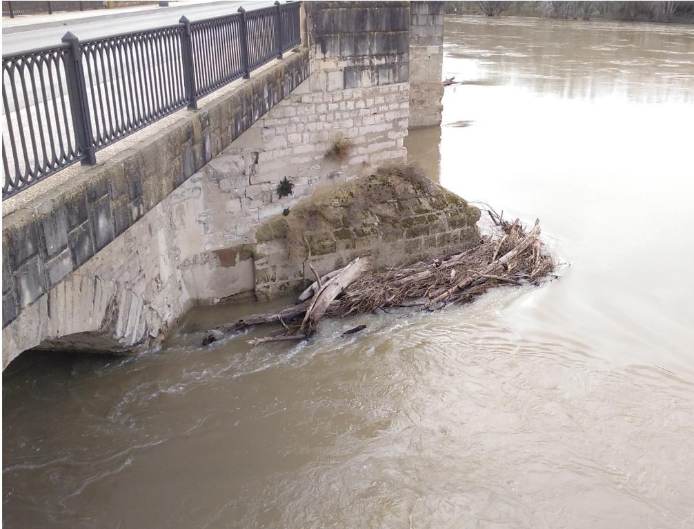
**Figure 2.** Example of debris accumulation around a bridge pier. River Ebro, Spain. Courtesy of Martin-Vide, J. P.
