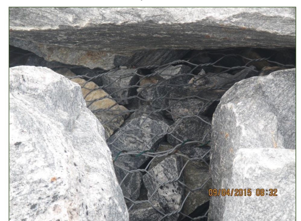
Inspection of Base of ASDS Groin
