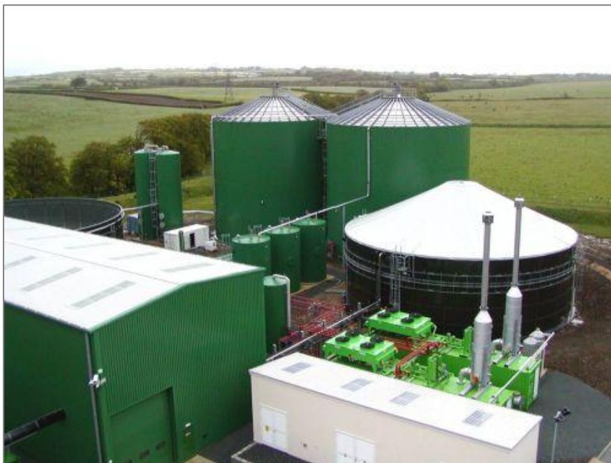
Holsworthy AD plant
