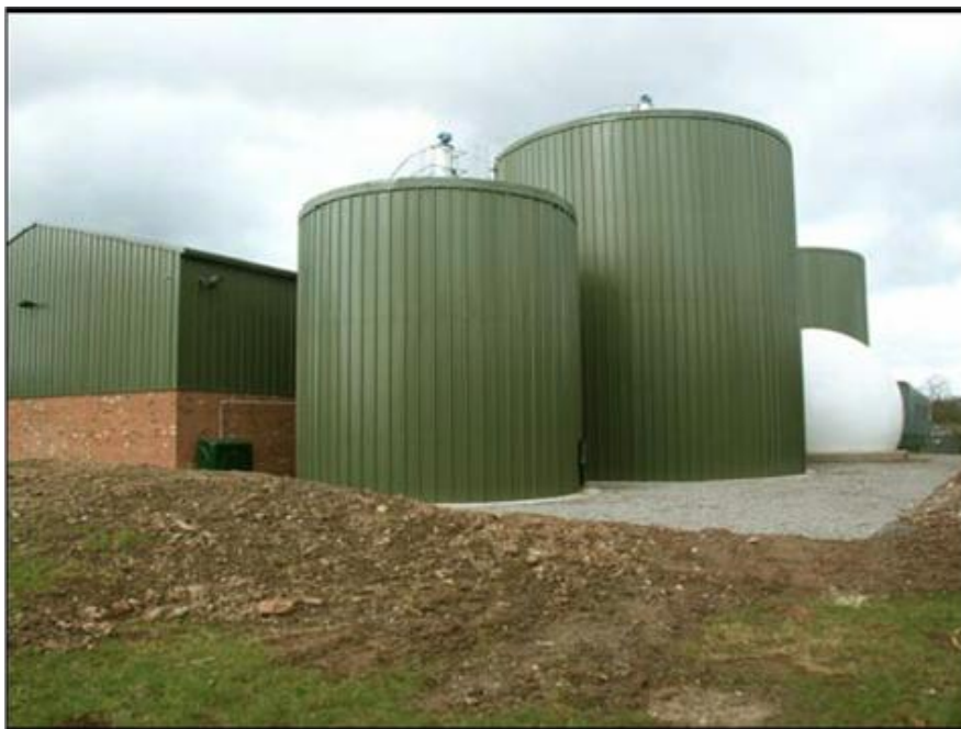
Digester under construction
